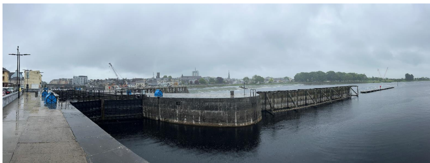
Photograph 4 – The control works in Athlone (23/05/25). Please note the waterways canal to the left, the sluice gates and 170m long overflow weir (background).
