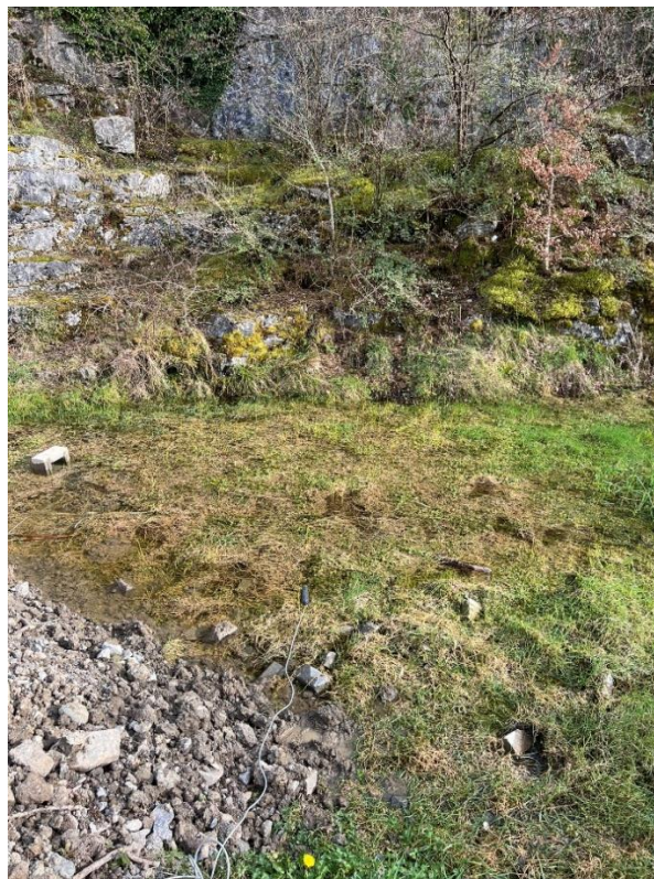
Photograph 3 –Sump located within the central part of the proposed outdoor theatre where surface water generated on site is ponding during heavy rainfall (24/03/25).
